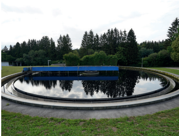
The Holzkirchen wastewater treatment plant is used for sampling in the project.
