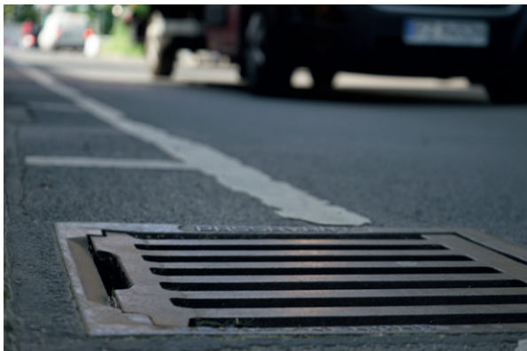
Tire debris entering through street drains is one of the sources of microplastics in the environment.
